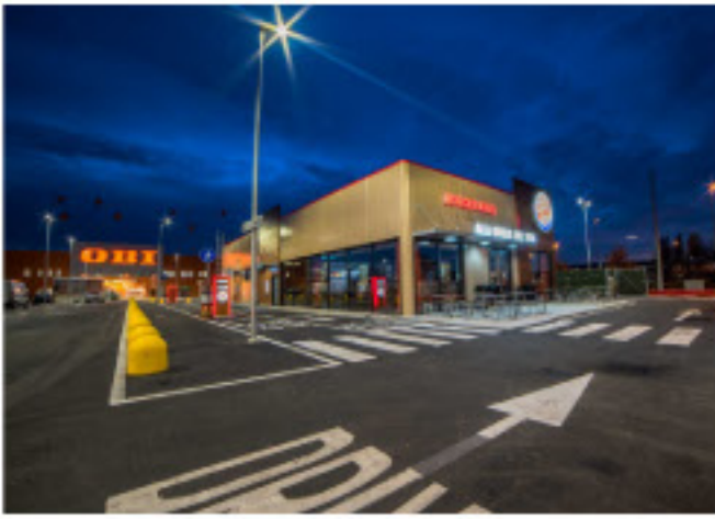
PUMPING SYSTEMS FOR THE OBI BURGER KING BUSINESS PARK
