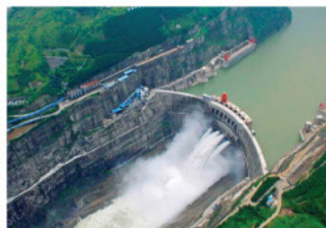
Xiluodu hydropower station
