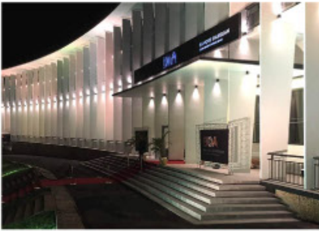
A FIRE-FIGHTING SET FOR THE NEW PREMISES OF ABIDJAN BANQUE IN COTE D'IVOIRE
