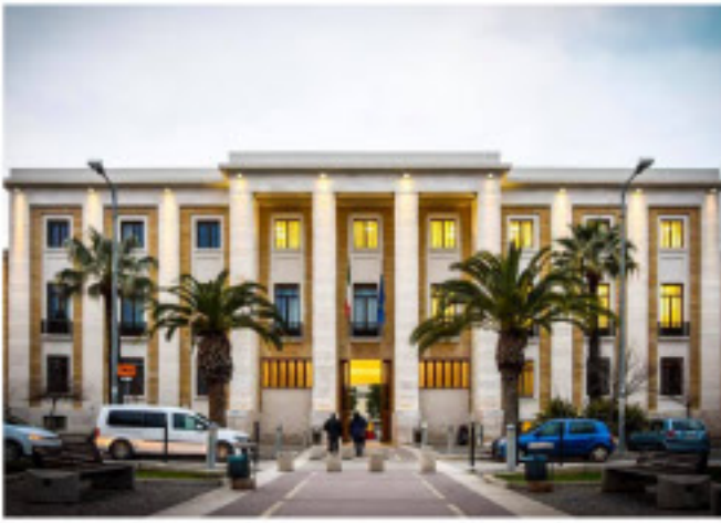
HEATING SYSTEM FOR THE POLYCLINIC OF BARI (ITALY)
