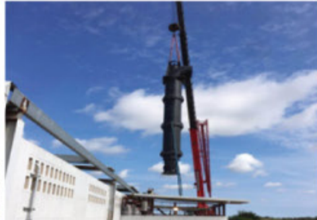
Texas flood control, USA
